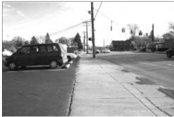
The lack of landscaping is apparent throughout the City's commercial district.
