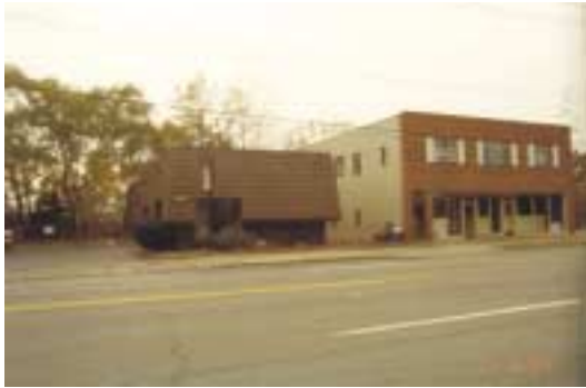
The absence of proper design standards can result in a lack of architectural harmony between buildings.
